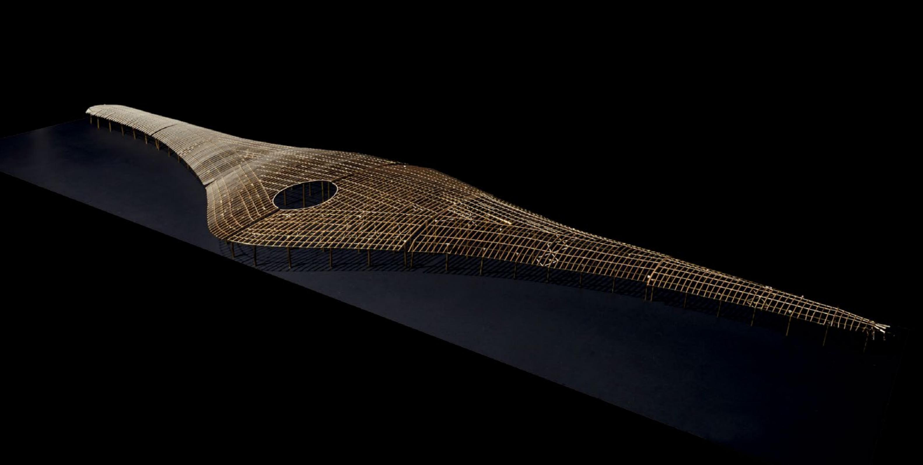
The design intent at Panama's Tocumen Airport was to create a series of long span beams that defined the gently curving form of the roof along the full length of the building. In order to avoid the substantial seismic loads of the region reaching the steel roof structure, a ductile 'fuse' for the top of the reinforced concrete columns was conceived and designed by the structural engineering team.
