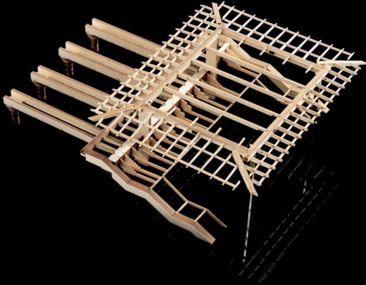
The central space is covered by a thin tapering roof that cantilevers approximately eight metres beyond the façade on each of the four sides. This structure is supported on only four steel columns to minimise the structure, while a mezzanine balcony cantilevers into the generous interior.
