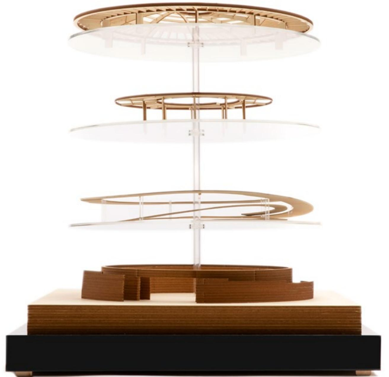
The structure of this new winery spirals up through the fermentation space to the top floor with panoramic views across the vineyards of the Le Dome Domaine. The roof is a structural timber dome where a central opening is created by rotating each of the roof beams. The circular structural geometry continues down through the volume to create a single cohesive building form.
