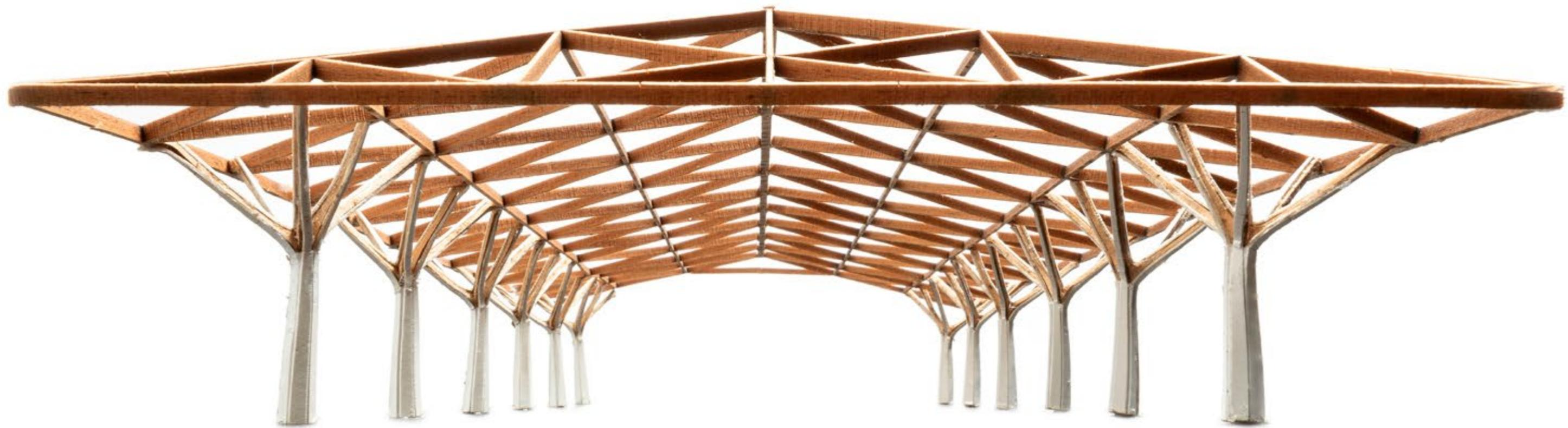
The roof structure of the new winery spans the 28 metres across the central space with a grid of beams that are three times shallower than what would be achieved with a classic beam system. The roof uses the pitched geometry to resist the applied loads through compression as well as bending. The supporting 'tree' structures provide both the vertical and lateral support to the roof.
