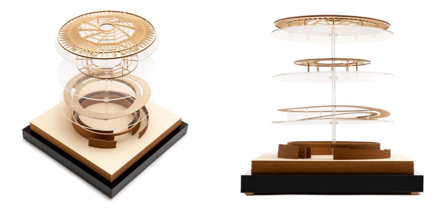
The structure of this new winery spirals up through the fermentation space to the top floor with panoramic views across the vineyards of the Le Dome Domaine. The roof is a structural timber dome where a central opening is created by rotating each of the roof beams. The circular structural geometry continues down through the volume to create a single cohesive building form.
