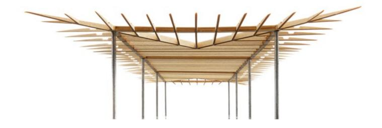
Conceived as a single element to provide shading beside the old port in Marseille, the detailing of this canopy is minimal. The perimeter is a single thin line, with the gutter set back inside the roof, with the canopy structure orientated to avoid an edge beam. Lateral stability is provided through frame action of the columns, which are fixed both at roof level and by the ground beams that connect the column bases.
