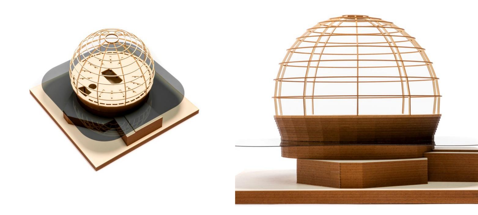
One of the unique features of this 30 metre dome structure is the structural interaction between the steel ribs and the glass panels. The glass panels provide bracing against buckling to the steel members, as well as stiffening the entire enclosure against lateral loads. The resulting steel structure is exceptionally small, with the ribs dimensioned at less than 1/200 of the dome span.
