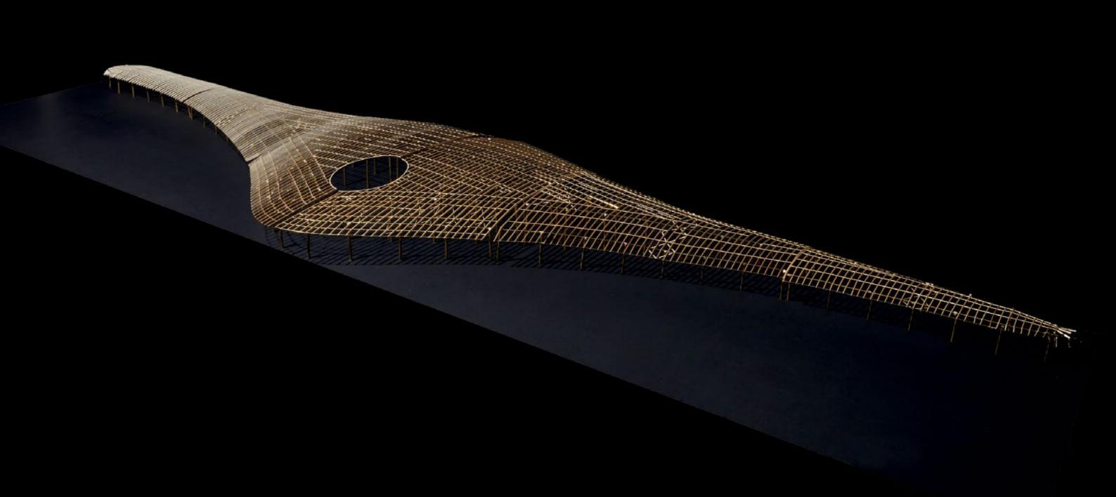
The design intent at Panama's Tocumen Airport was to create a series of long span beams that defined the gently curving form of the roof along the full length of the building. In order to avoid the substantial seismic loads of the region reaching the steel roof structure, a ductile 'fuse' for the top of the reinforced concrete columns was conceived and designed by the structural engineering team.
