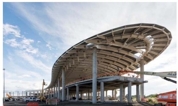
Figure 8. Tocumen Airport recent site progress
