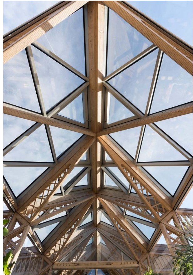
Figure 13. Maggie’s Centre Roof
